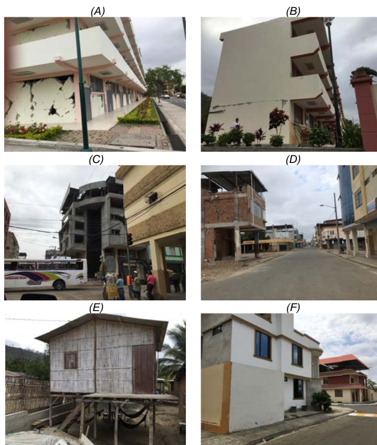
Fig. 4: Examples of building styles and damage in Portoviejo. (A) and (B) are the same style of construction but suffered much more, and less extensive damage respectively, perhaps related to the underlying geology. (C) is a damaged precast concrete slab building in the central business district (CBD), and (D) is a typical brick building in the CBD. (E) is a bamboo house typical of the suburbs. A new wall comprising concrete blocks and reinforcing steel for a concrete column is at left. (F) is a multi-story concrete slab building in a recent subdivision that was undamaged.
